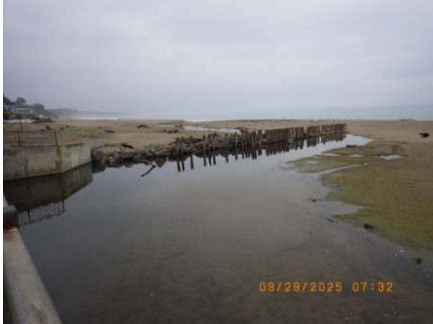
Looking southeast and downstream with the main Aptos Lagoon on the right and a sand berm at the end of the rock jetty, sealing off the freshwater lagoon from the outlet channel to the left of the jetty. 9-29-2025
