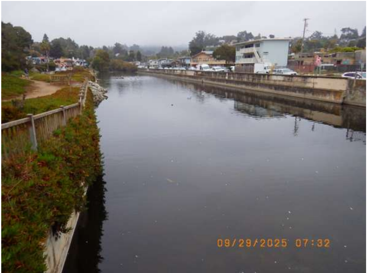
Looking north and upstream from the walk bridge at the leveed Aptos Lagoon. 9-29-2025
